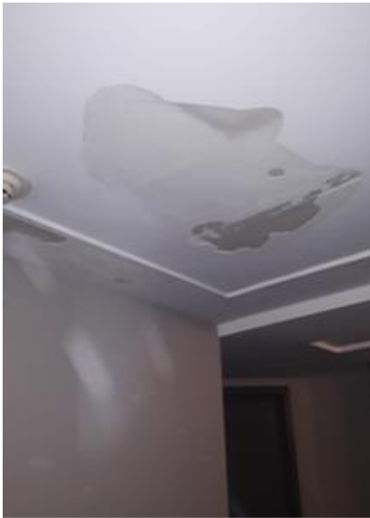
19 th floor ceiling repair
